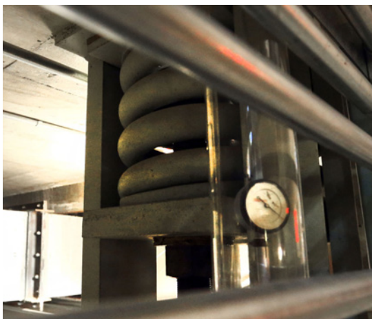
The Anechoic and Reverberant rooms rest
